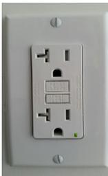
Ground Fault Circuit Interrupter (GFCI) outlet constantly monitors electricity flowing in a circuit to protect you from electrical shock in the event of a surge or water contact.
